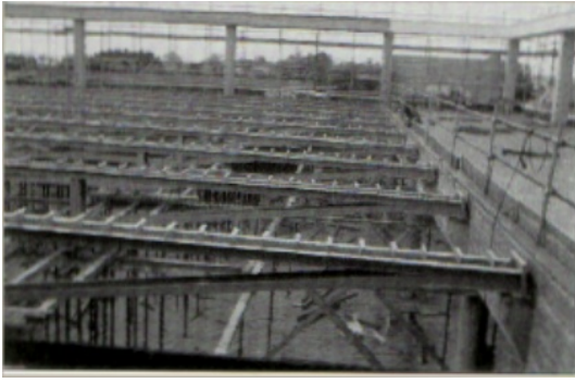
Figure 11. Detail of the roof cover of the Gulliver commercial center.
