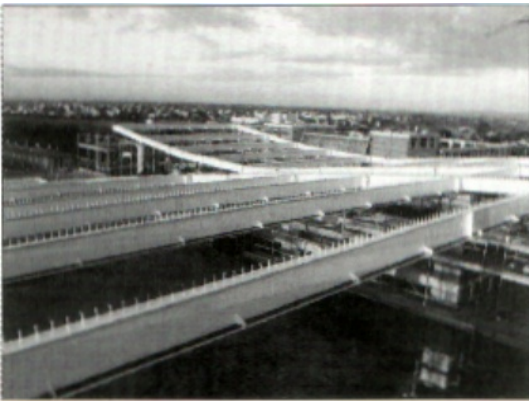
Figure 12. View of the roof cover of the La Lucchina multiplex.
