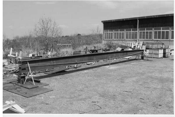
Figure 13. View of the girder.
