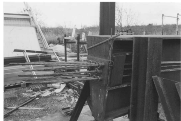
Figure 15. Anchoring the ends.
